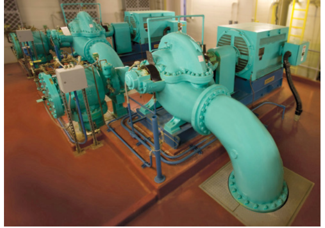
Boiler feed pumps
